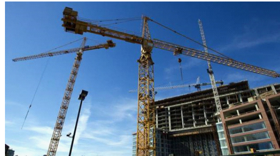
Cranes operate at a condominium construction site in Vancouver. Source: Bloomberg
