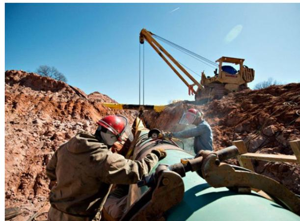
Welders secure a joint between two sections of pipe near Prague, Ok. Source: Bloomberg
